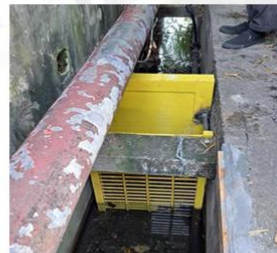
Install resin grease trap at end outlet of drainage
