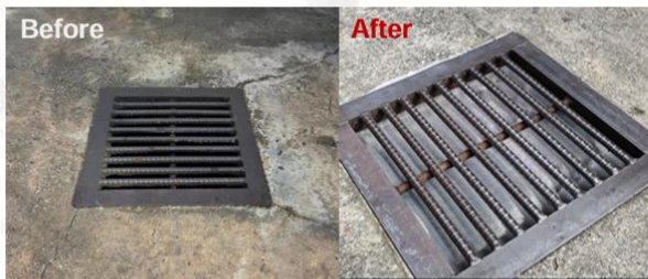
Install aluminium screen as drain filter to prevent resin flow into drain
